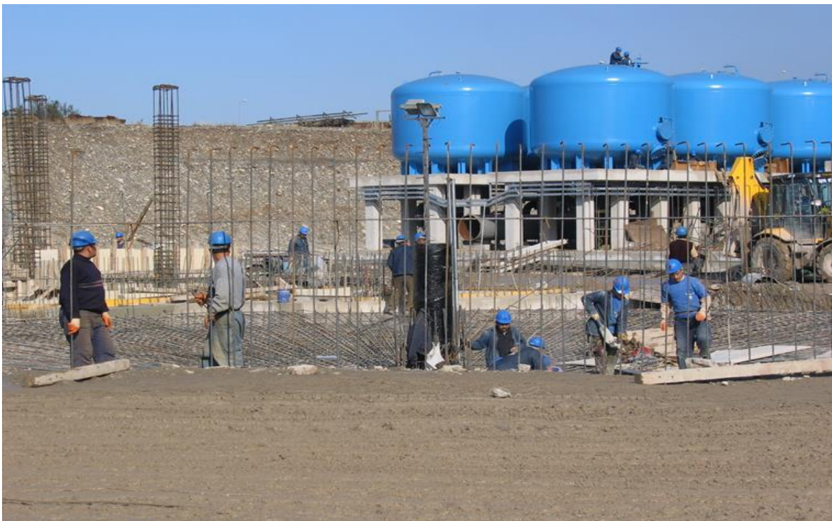
Sludge Thickener Area Construction
