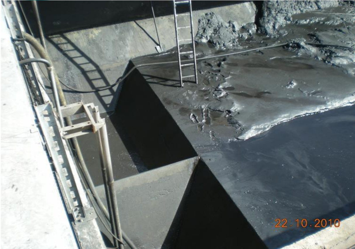
Settling Basin Sludge
