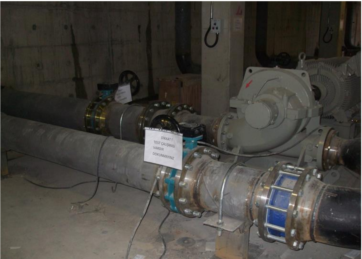
Pump Piping Installation
