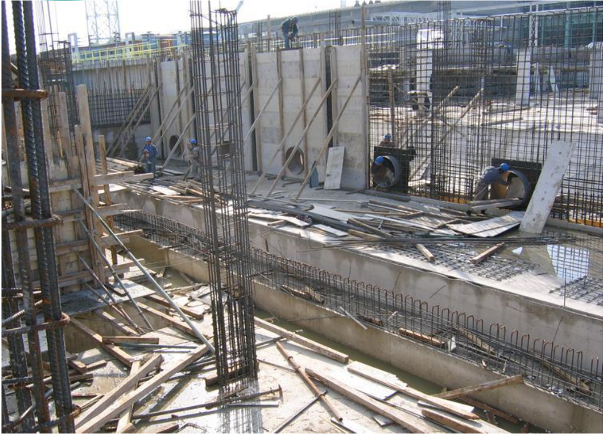
Cooling Tower Basin / Pump Suction Embedded Plate
