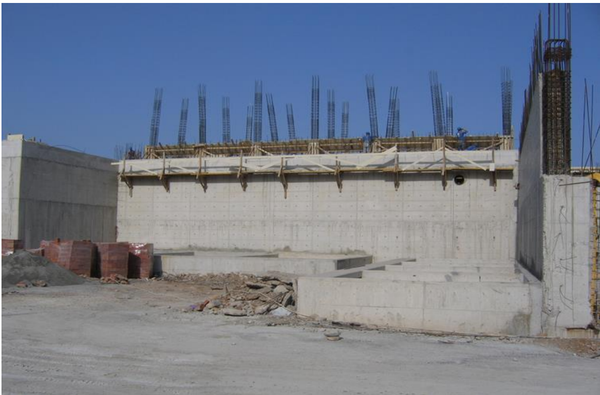
Chemical Dosing Units Construction
