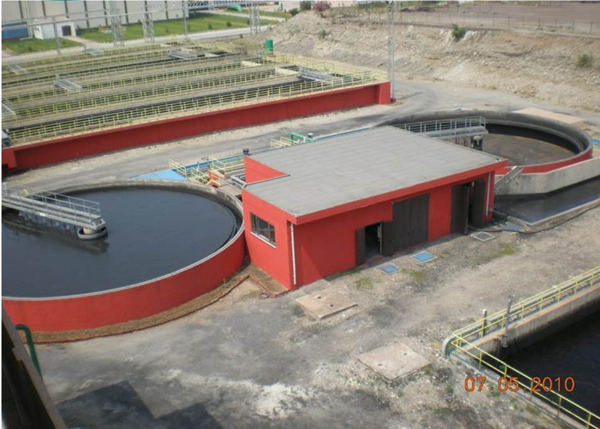
Sludge Thickener Area General Appearance
