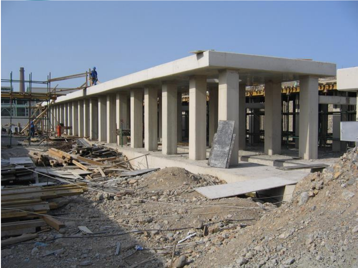
Sand Filter Area Construction
