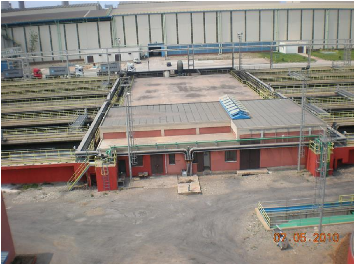
Settling Basin Area General Appearance
