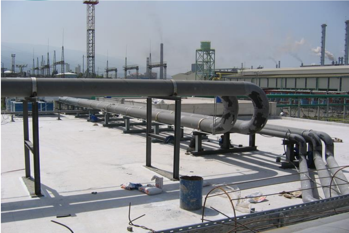
Pump Piping Installation
