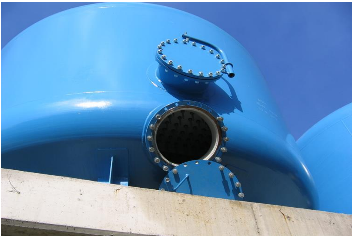
Sand Filter Bottom Side (Under Nozzles)
