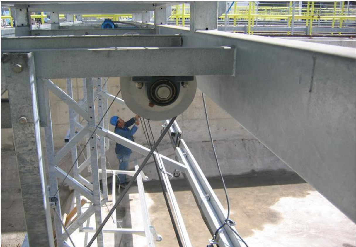
Settling Basin Scraper Bridge Installation
