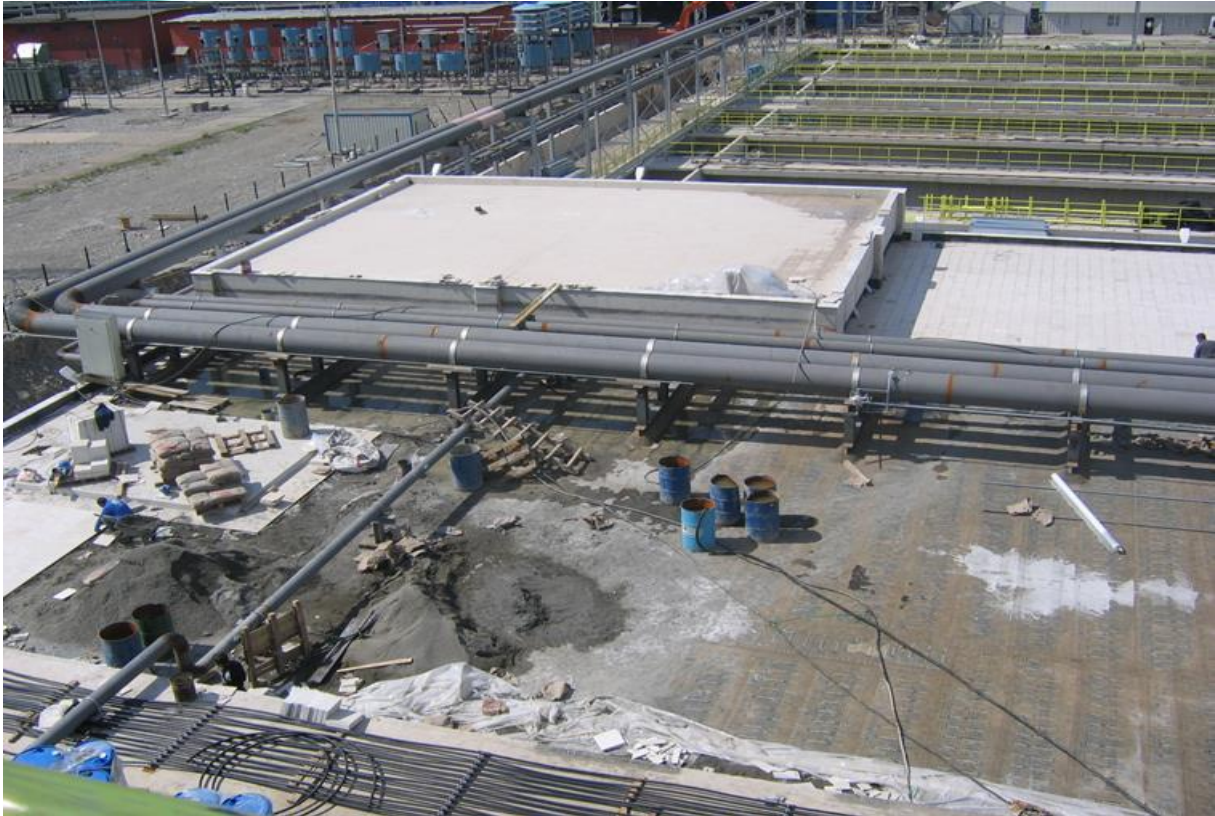
Pump Piping and Chemical Dosing Unit Piping Installation
