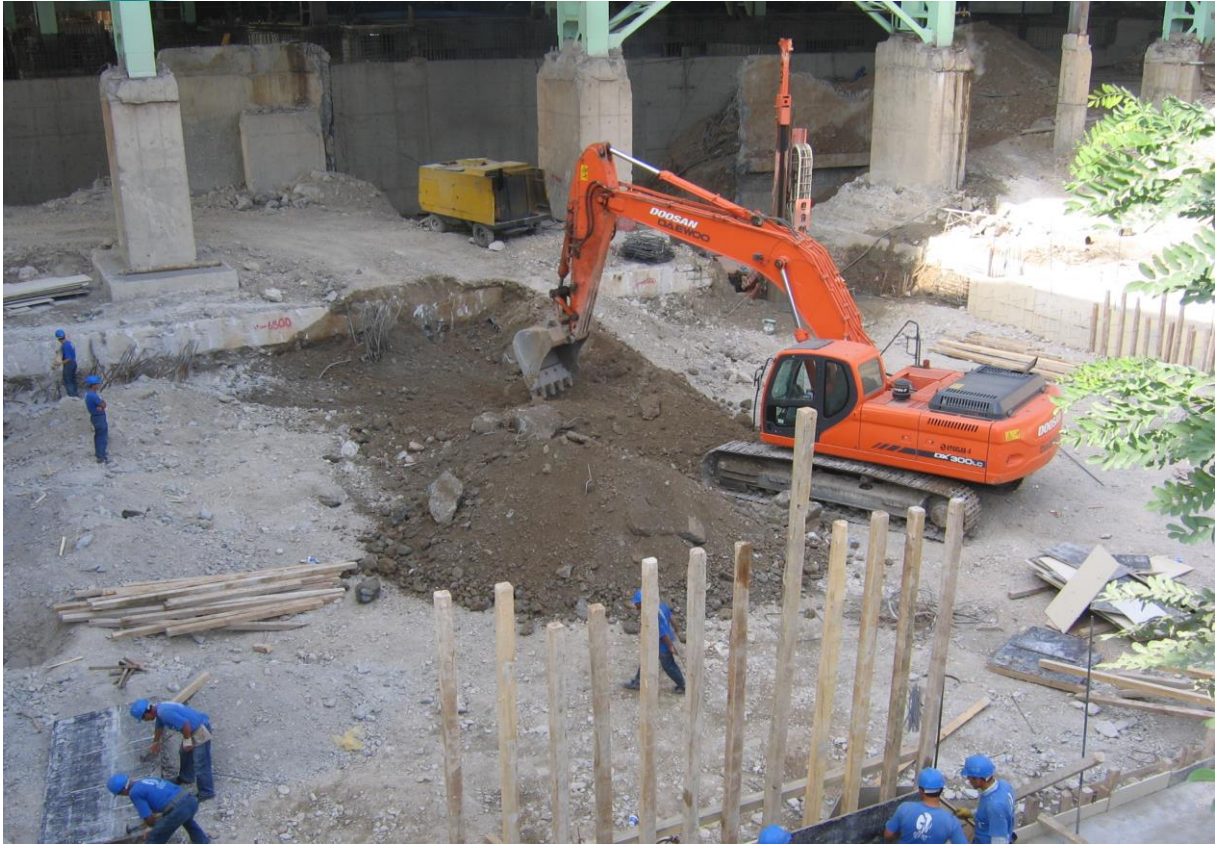
Scale Pit Excavation Work
