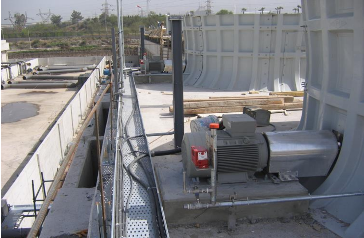
Cooling Towers Installation
