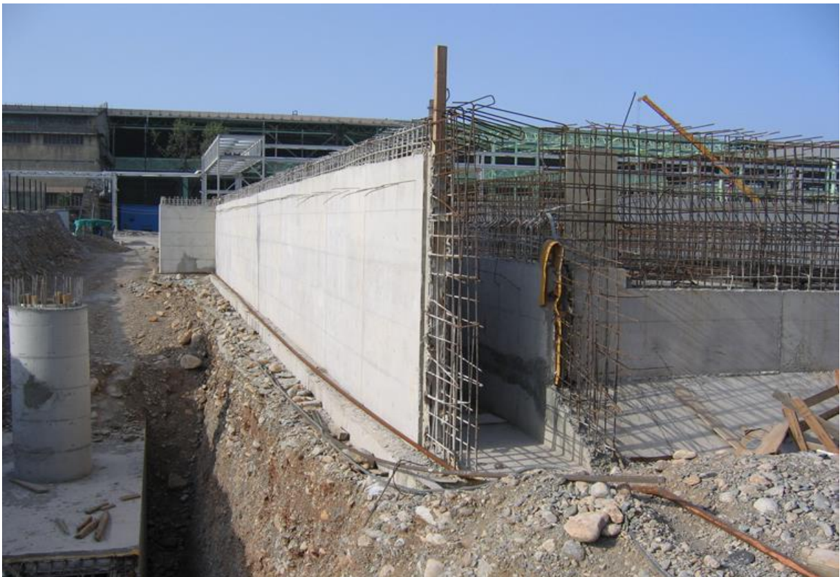
Settling Basin - Without Oil and Scale Water Basin ,Construction
