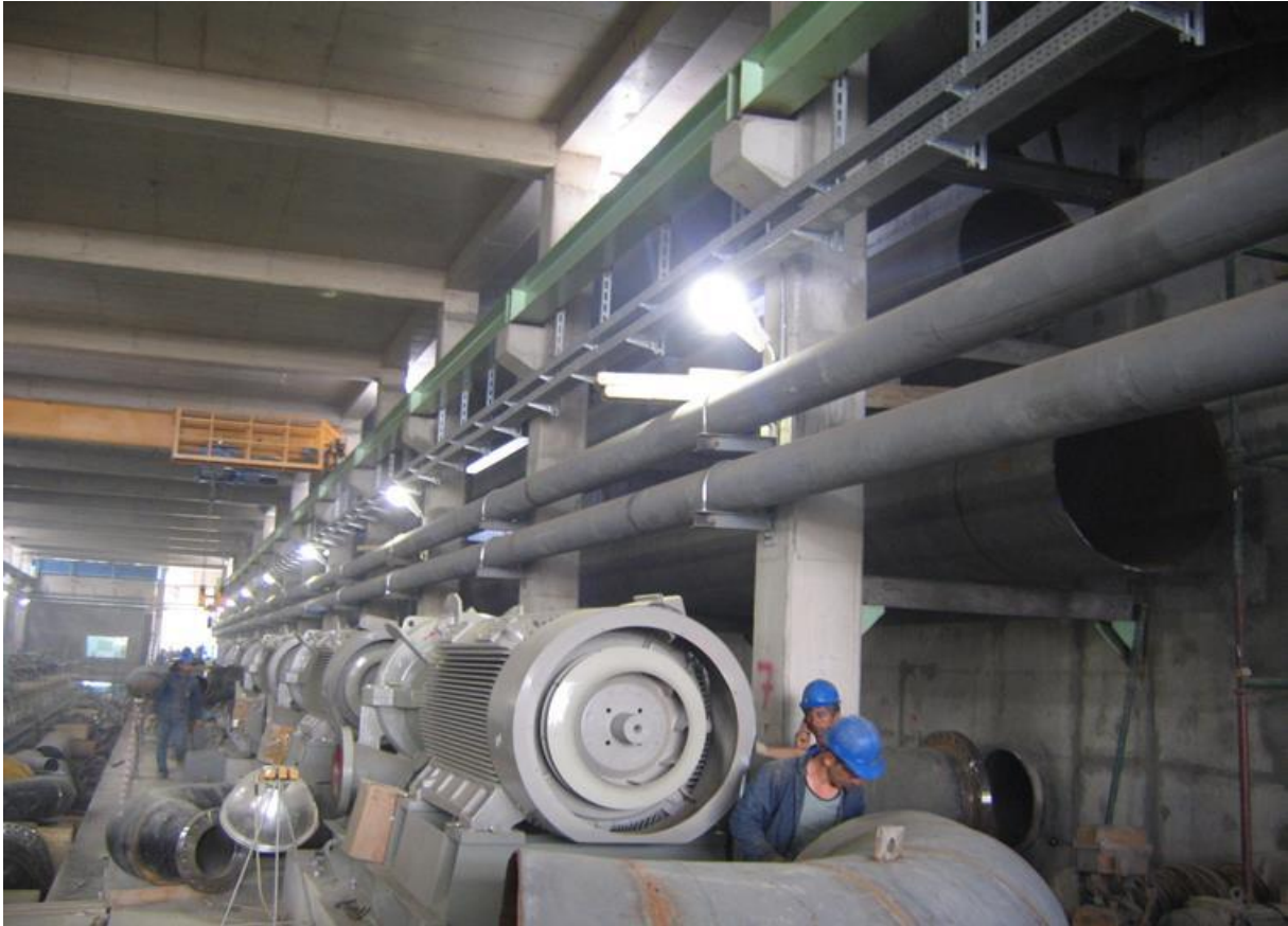
Pump Hall Piping Installation
