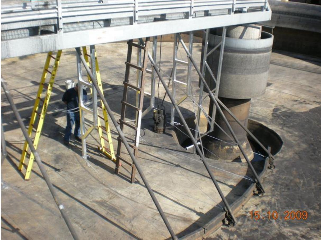
Sludge Thickener Bridge
