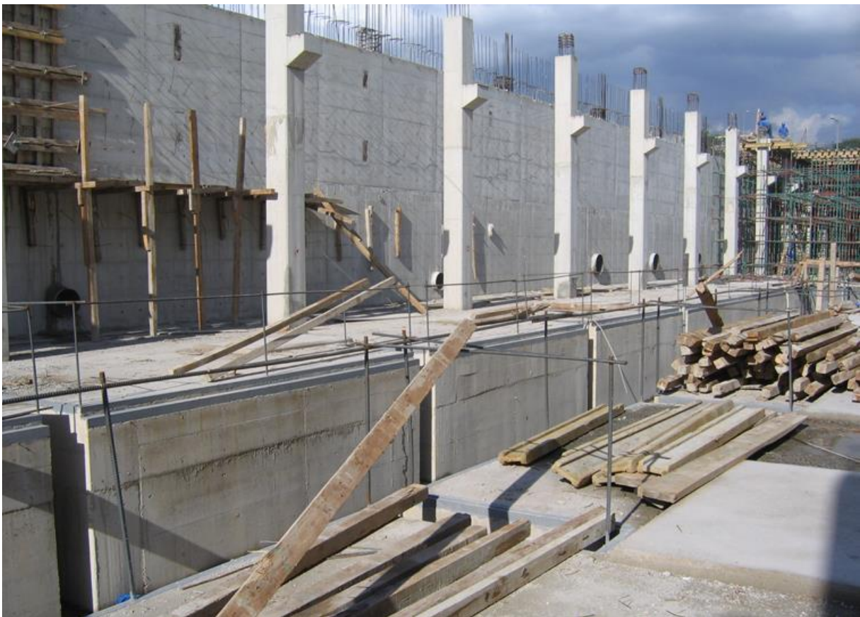
Cooling Tower Basin / Pump Hall Construction
