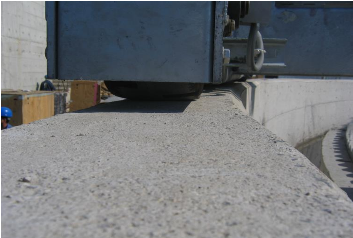
Sludge Thickener Bridge
