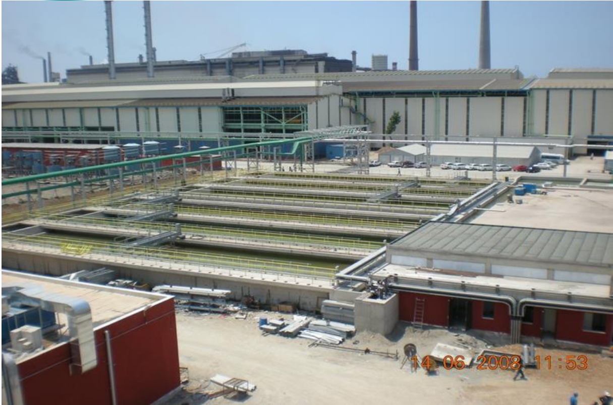
Settling Basin Area General Appearance
