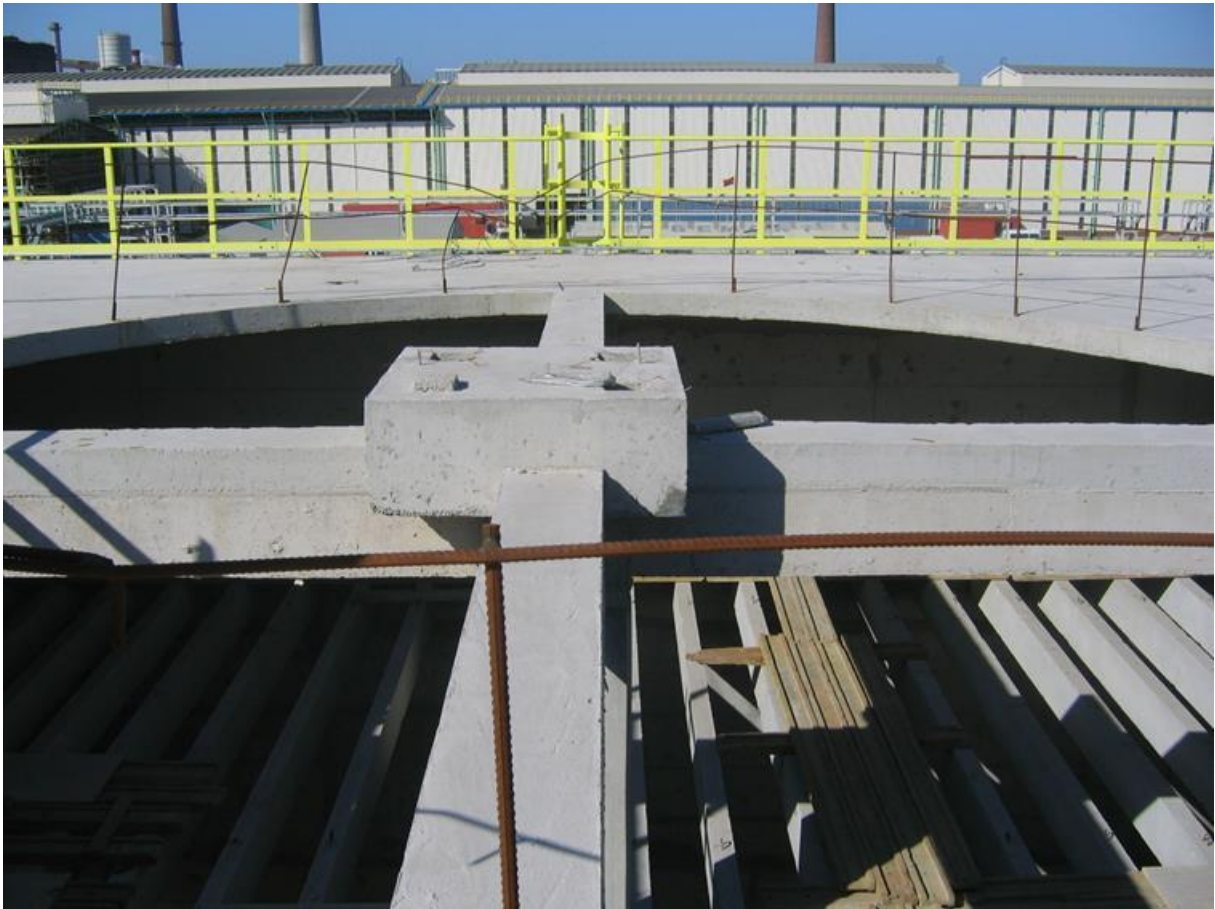
Cooling Towers Installation
