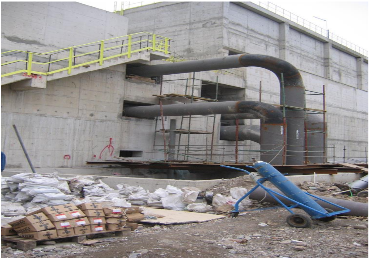
Pump Piping Installation
