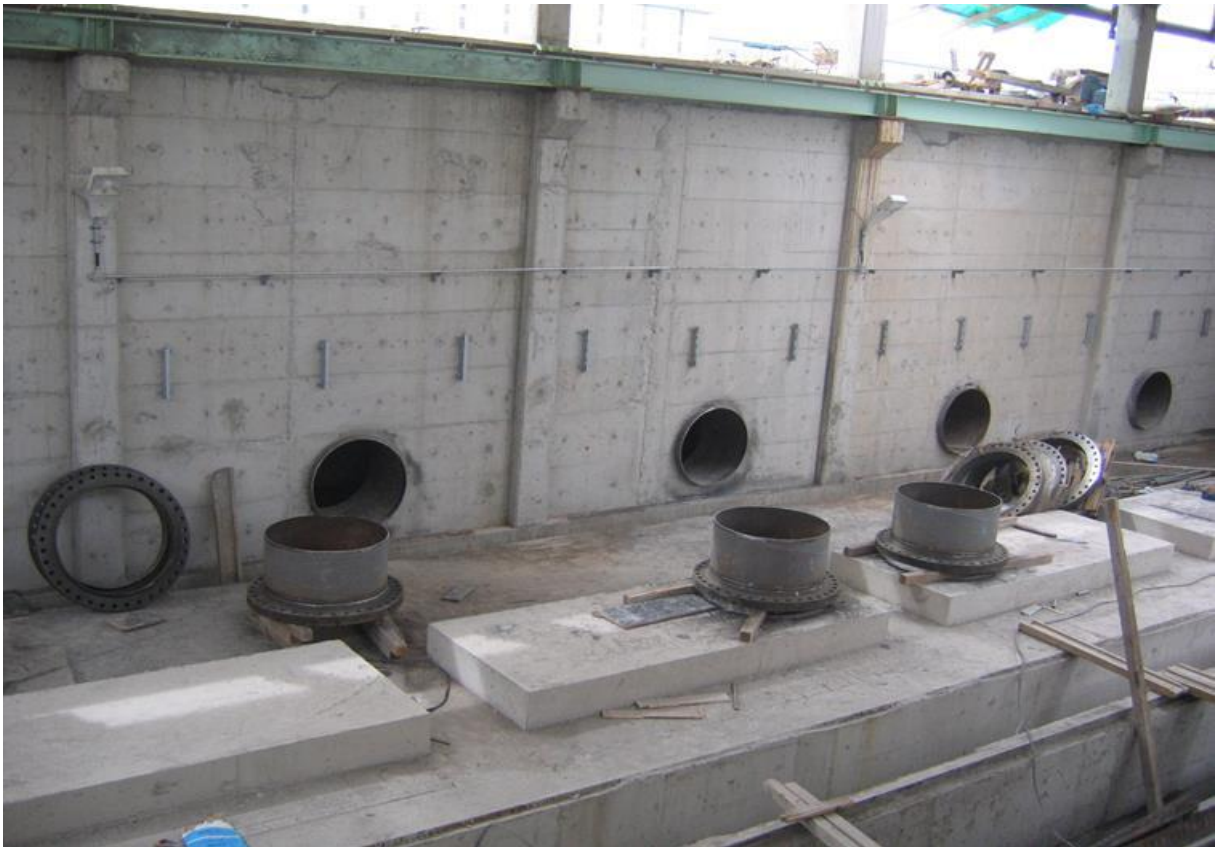
Pump Concrete and Suction Line
