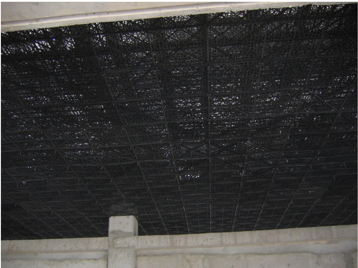
Cooling Towers Inside Grid Springing Installation
