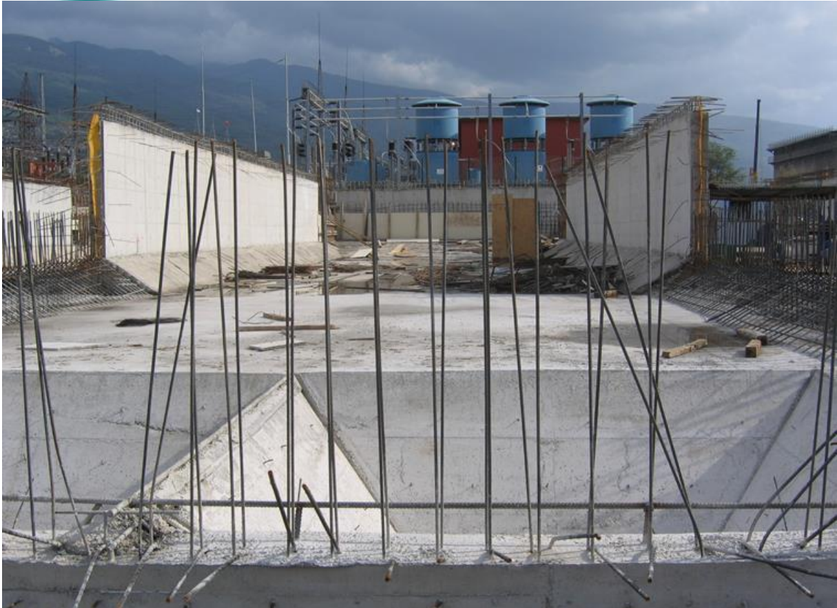
Settling Basin Construction
