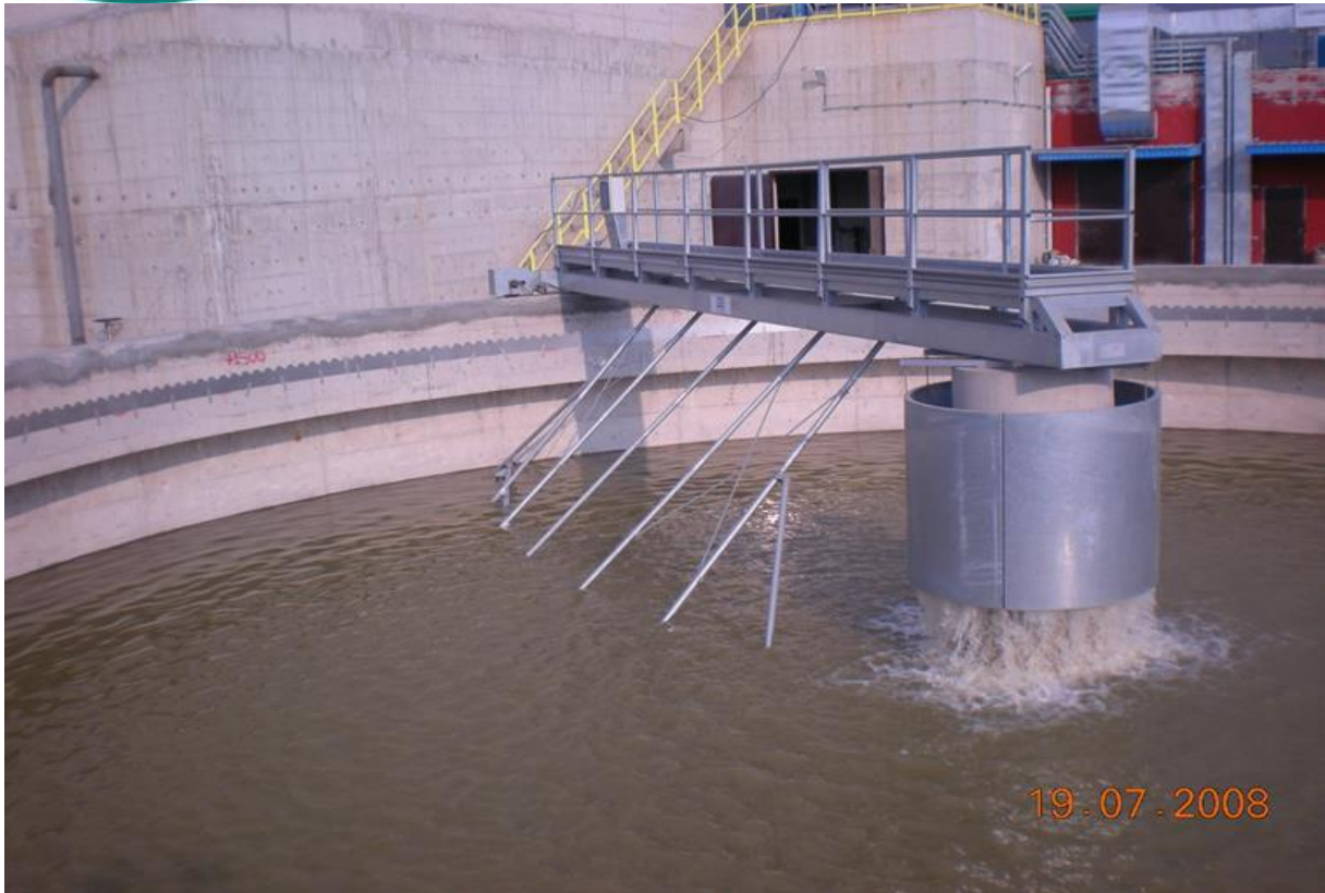
Sludge Thickener Bridge
