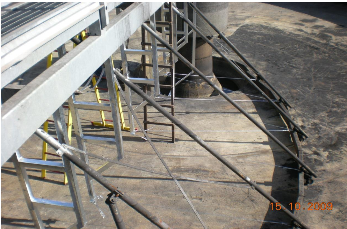
Sludge Thickener Bridge
