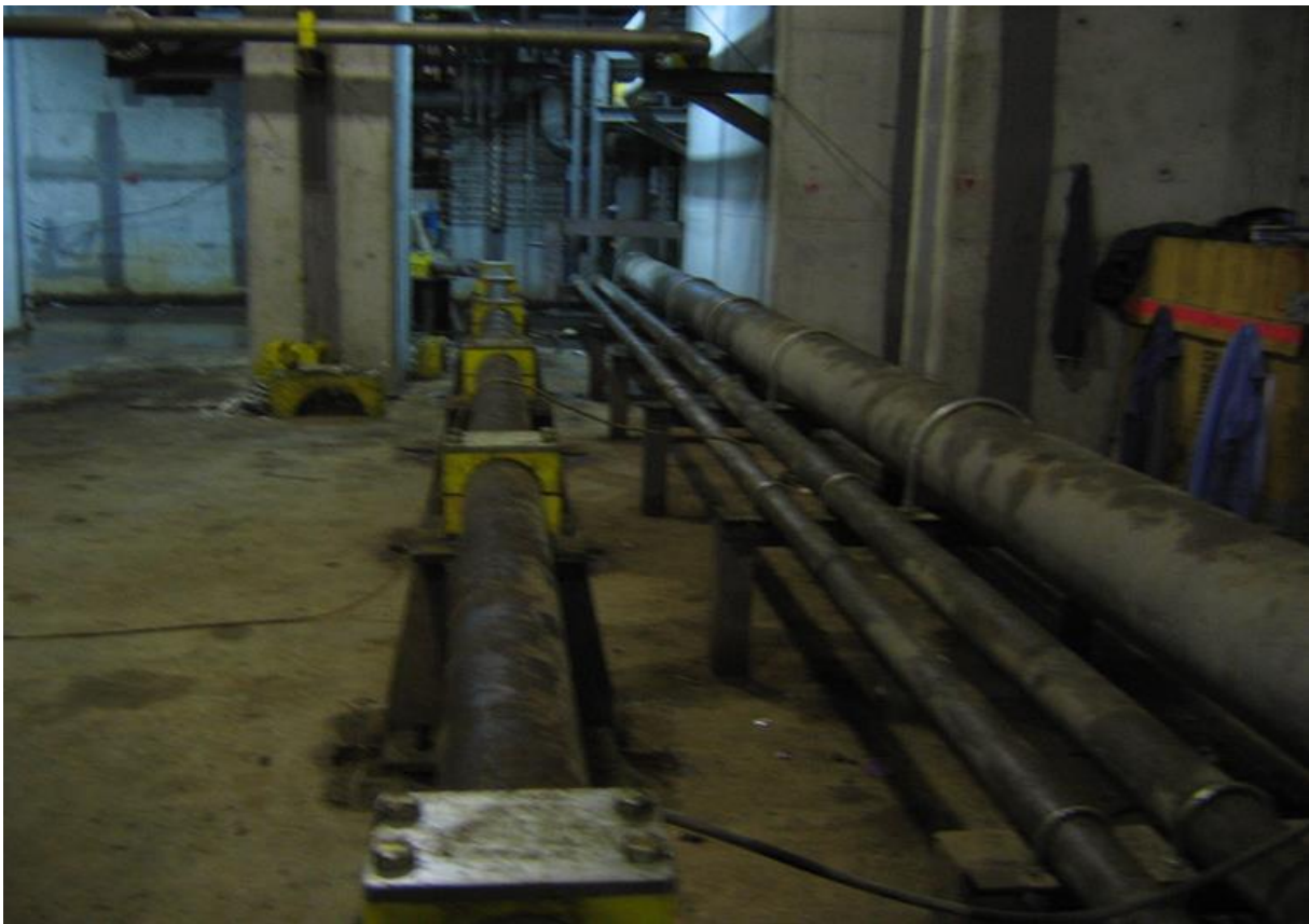
Descale Pump Discharge Line General Appearance
