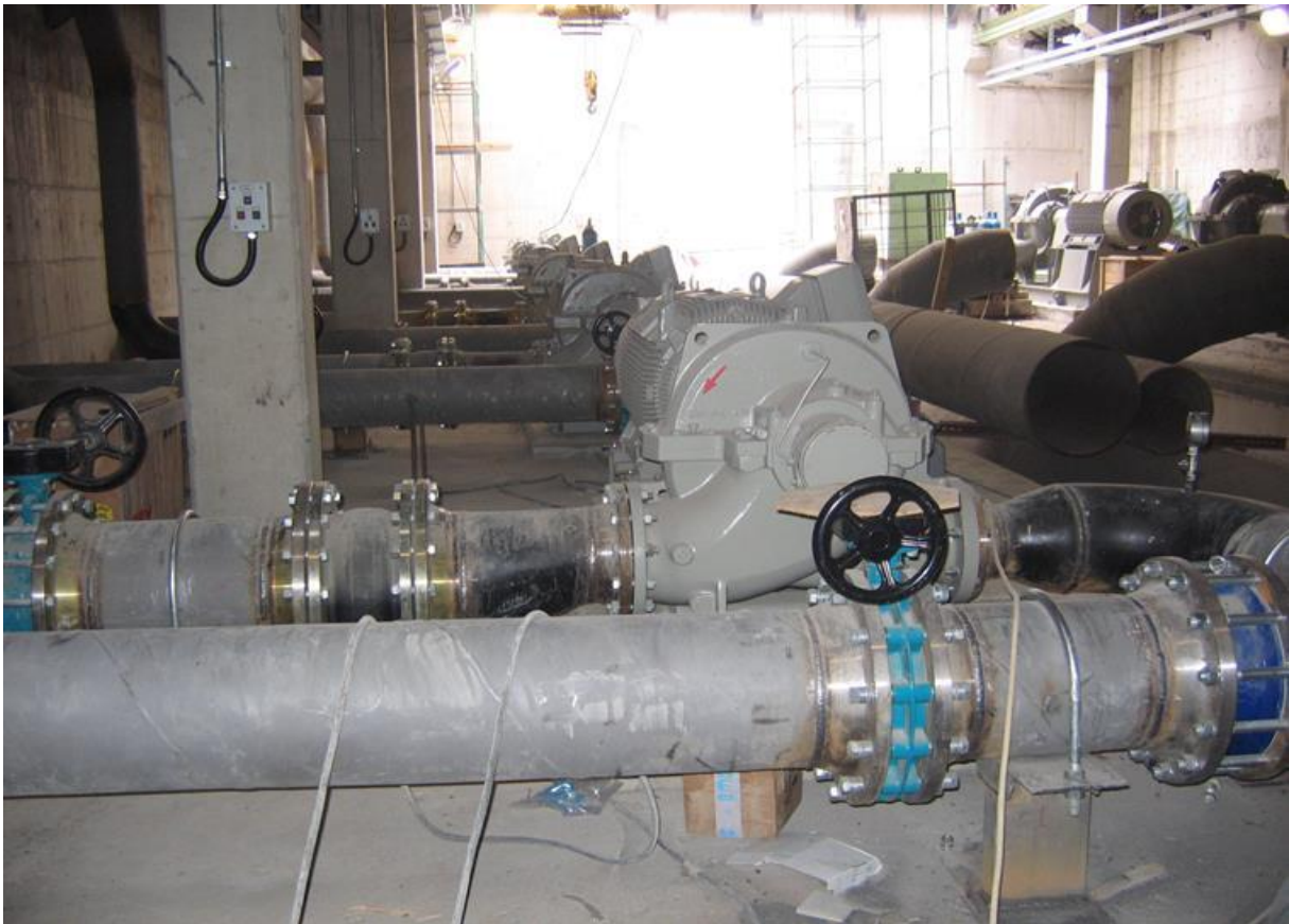
Pump Piping Installation
