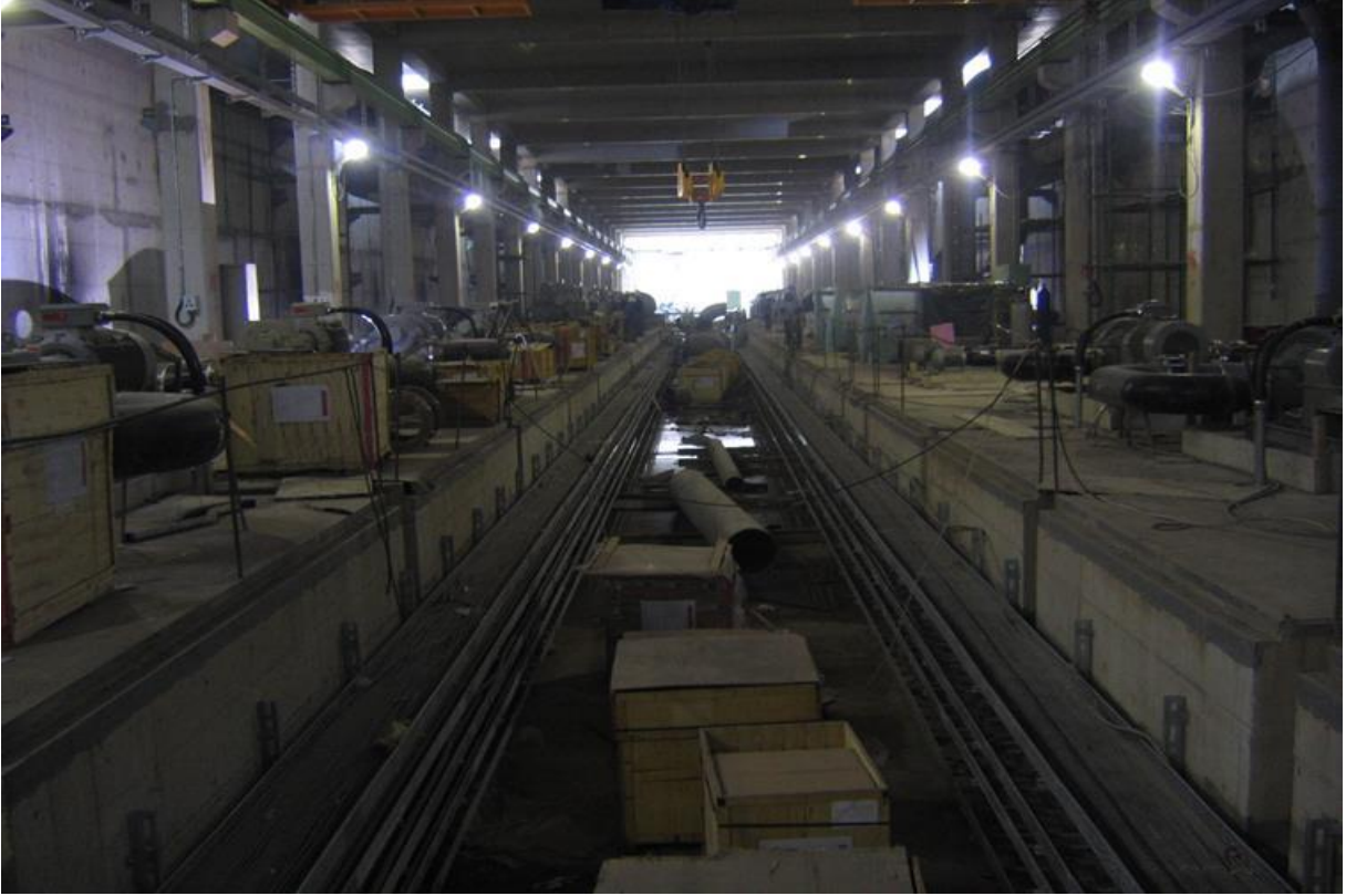
Pump Hall Piping Installation
