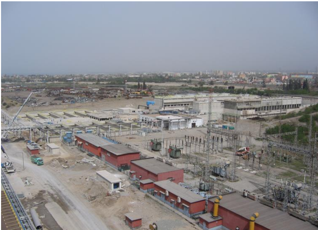
Water Treatment Plant General Appearance
