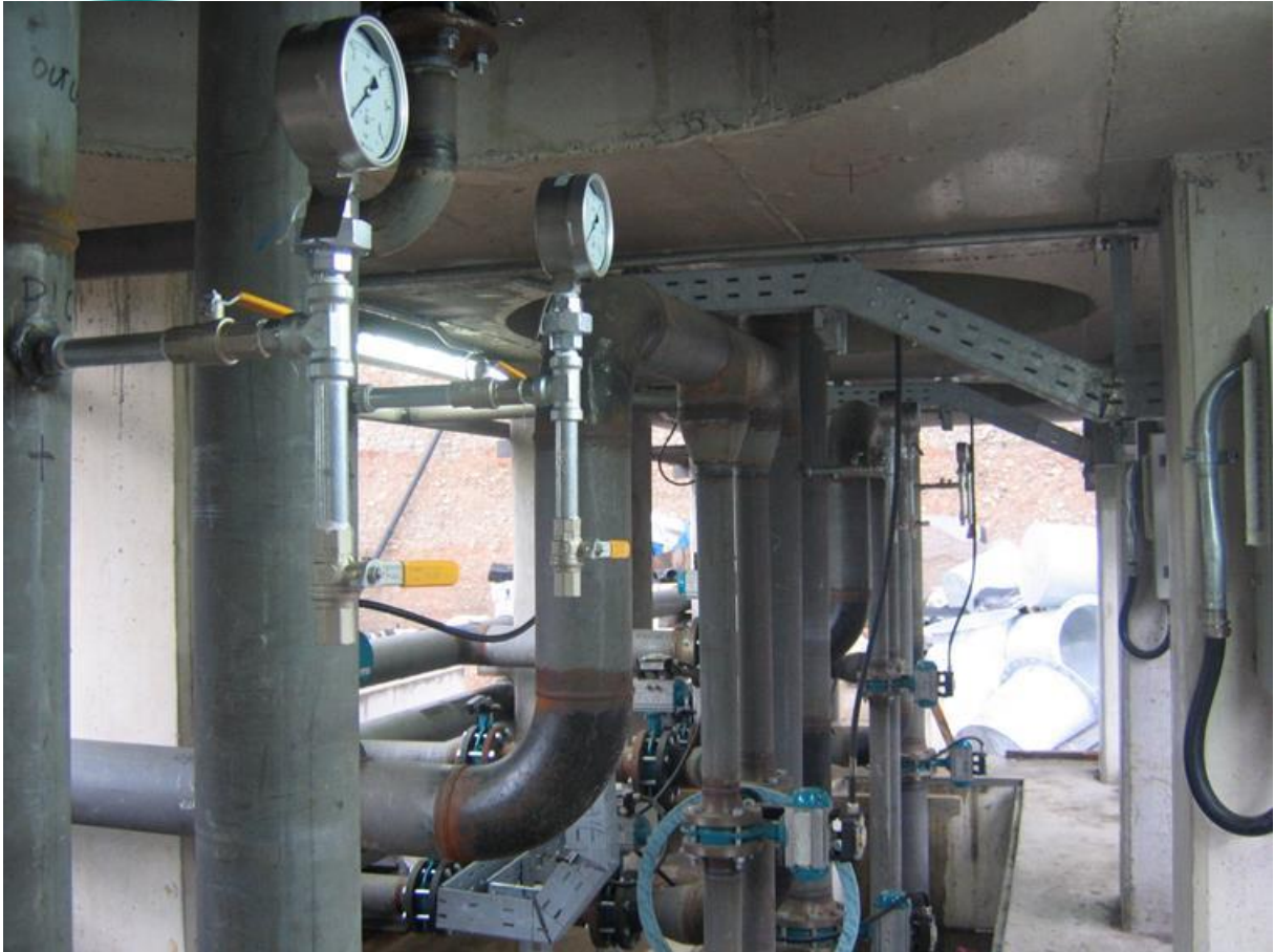
Sand Filter Valve Skid Area Installation
