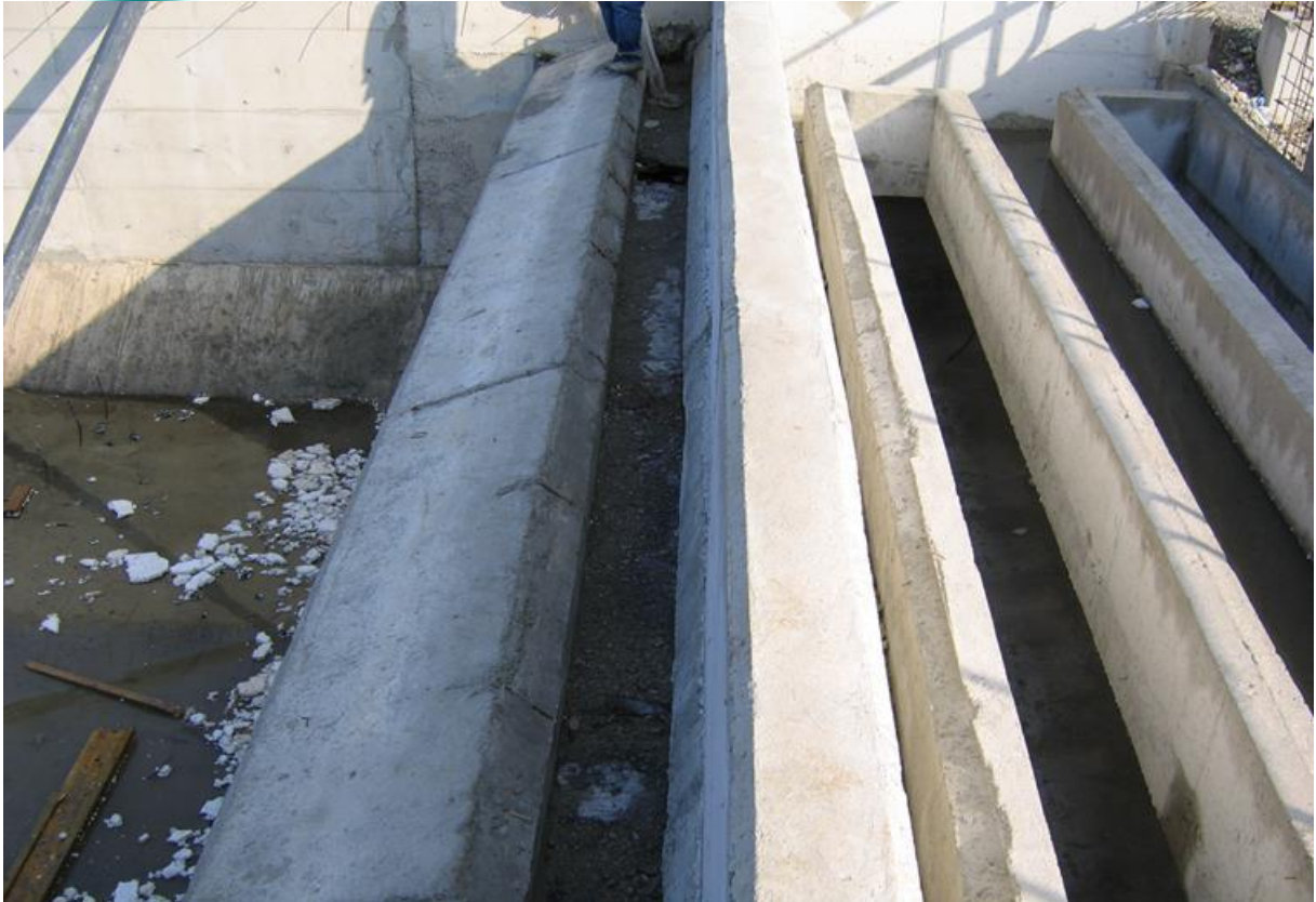
Settling Basin Oil Blade Construction
