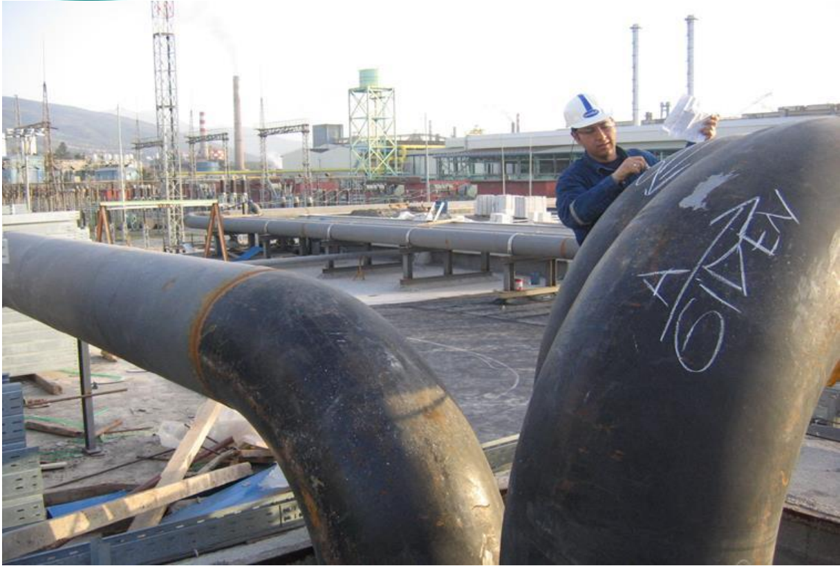
Pump Piping Installation
