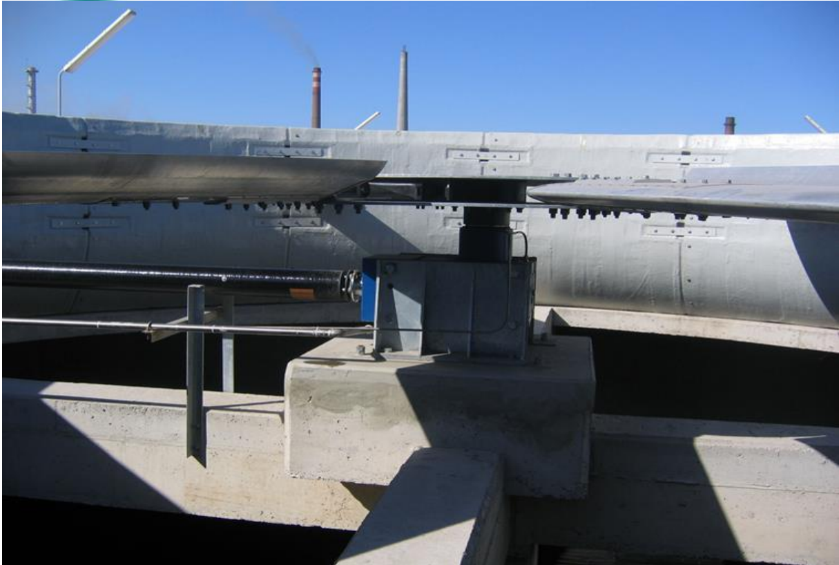
Cooling Towers Fan Installation
