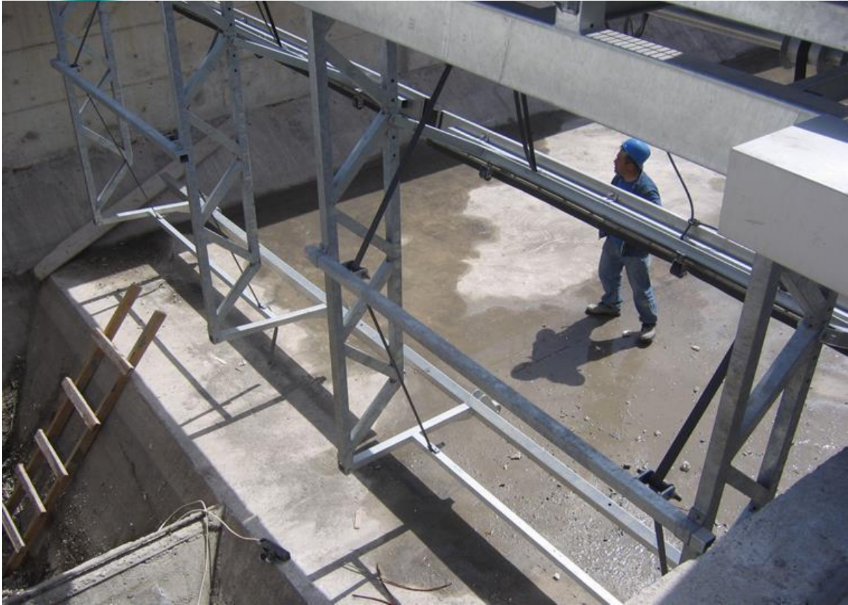
Settling Basin Scraper Bridge Installation
