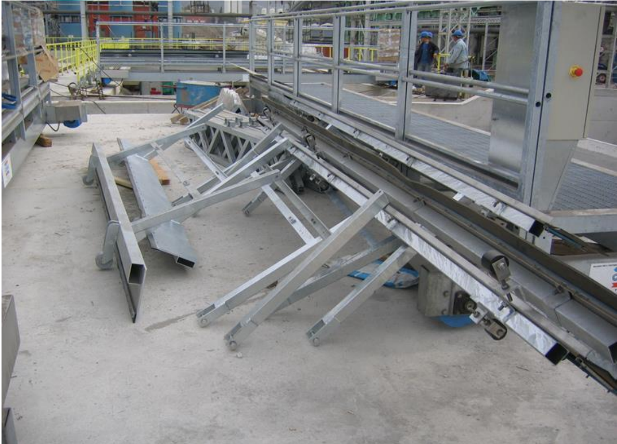
Settling Basin Scraper Bridge Installation
