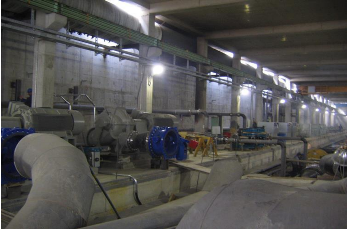
Pump Hall Piping Installation
