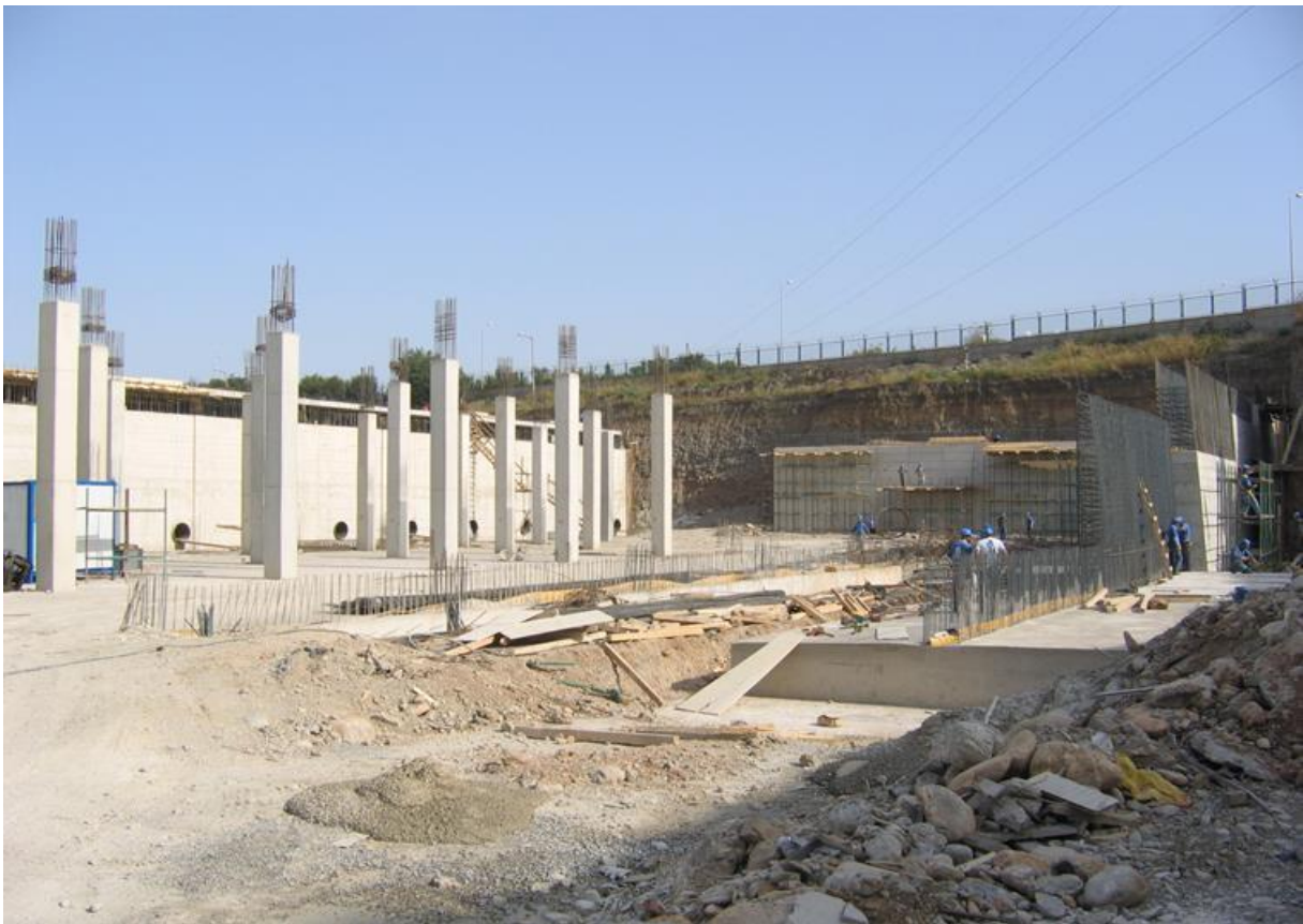
Cooling Towers Basin Construction
