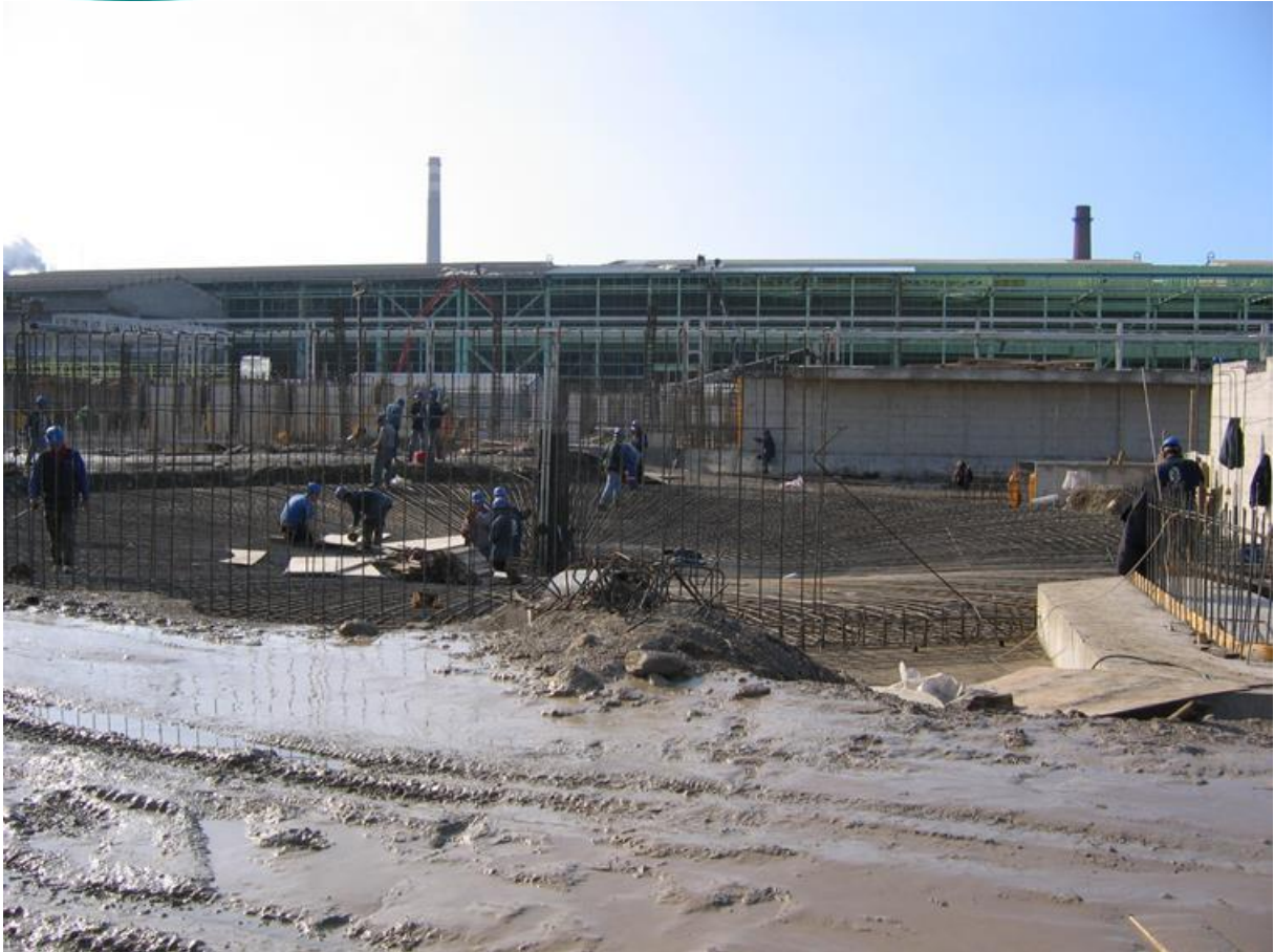
Sludge Thickener Area Construction
