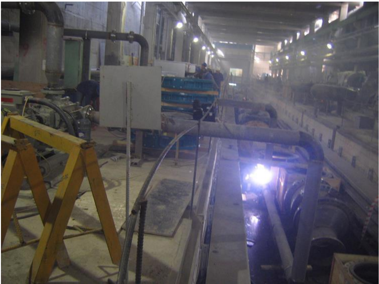
Pump Hall Piping Installation
