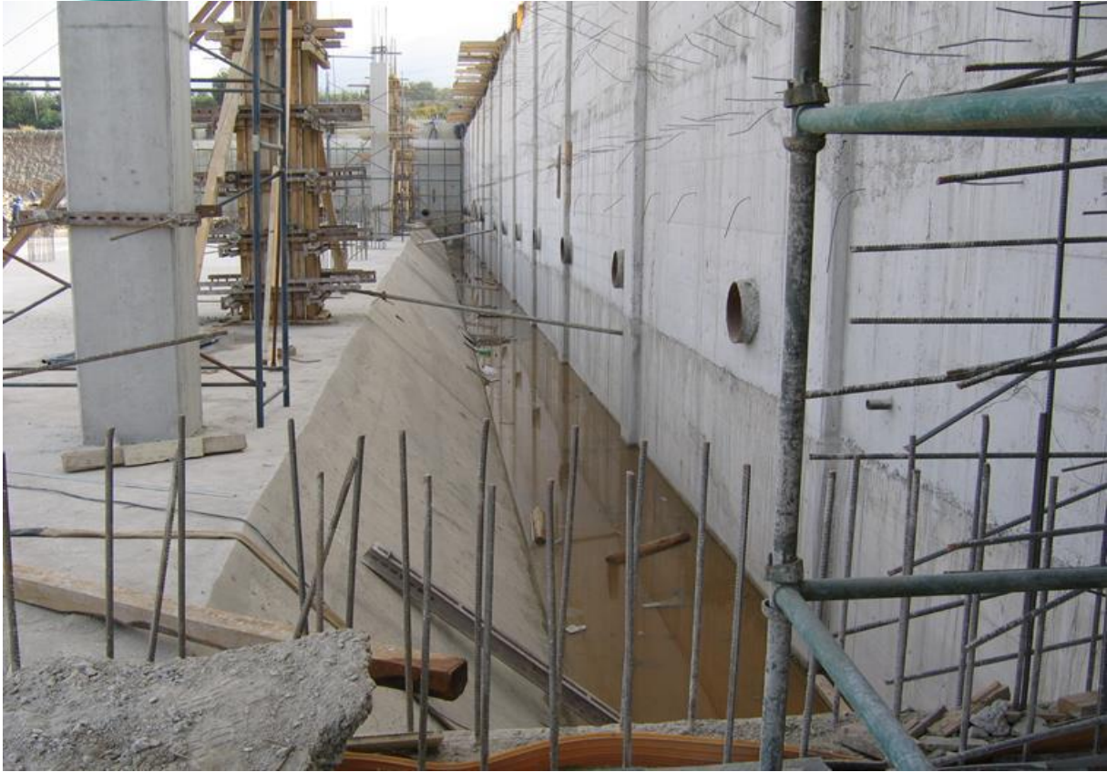
Cooling Tower Basin / Pump Suction Pit Construction
