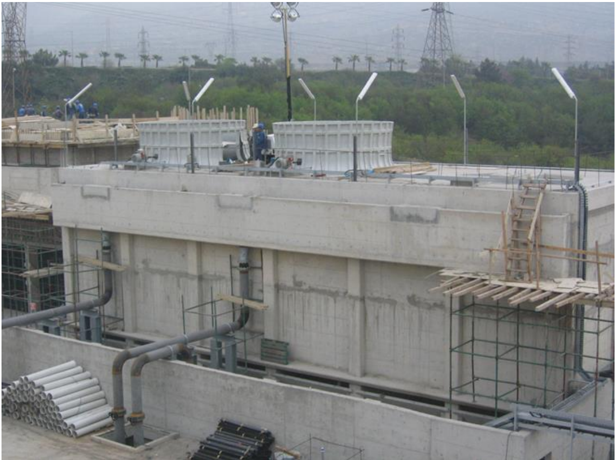
Cooling Towers Installation
