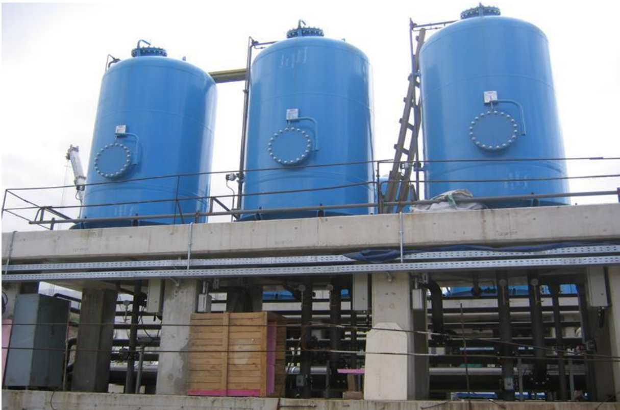
Sand Filter Area Installation
