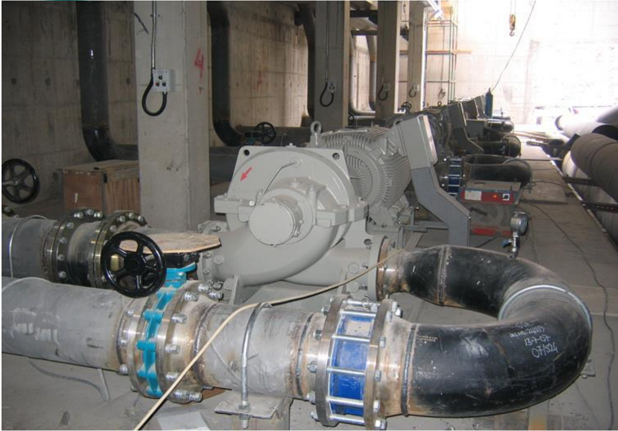
Pump Piping Installation
