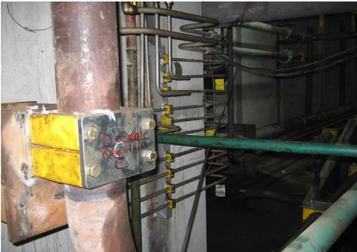
Descale Pump Dicharge Line Generel Appearance
