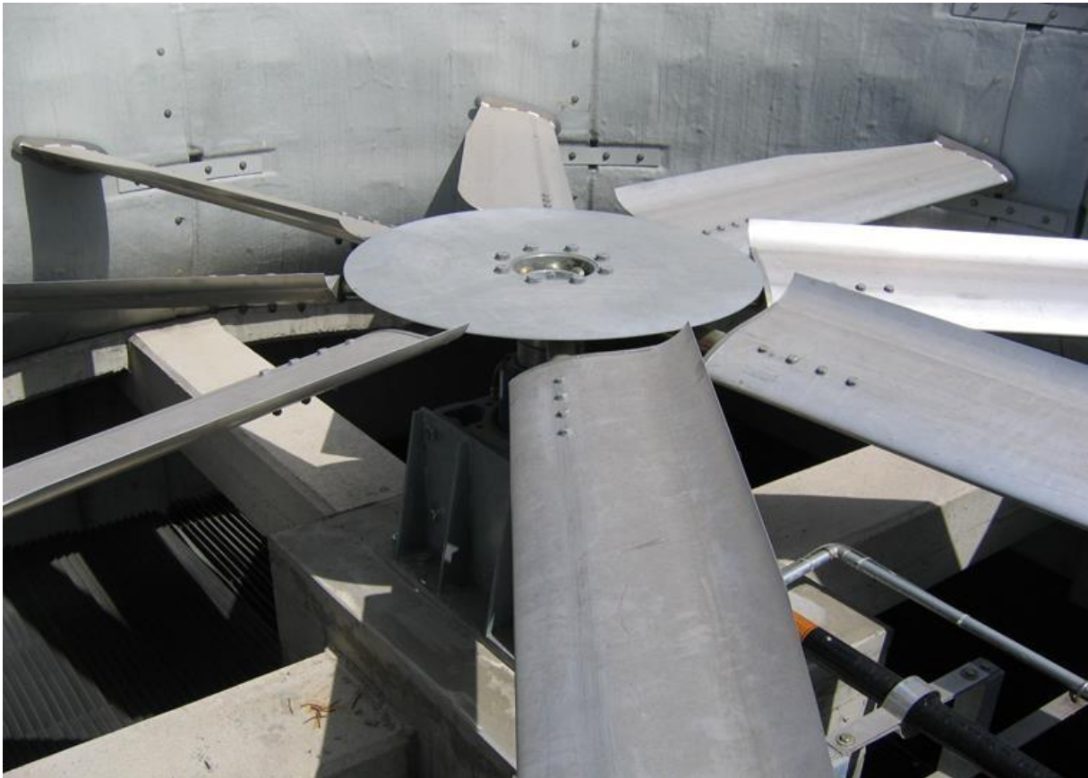
Cooling Towers Fan Installation
