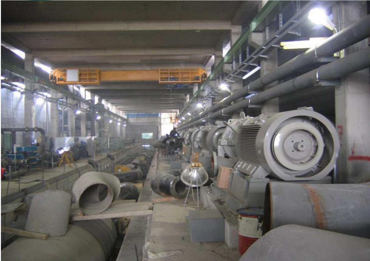
Pump Hall Piping Installation
