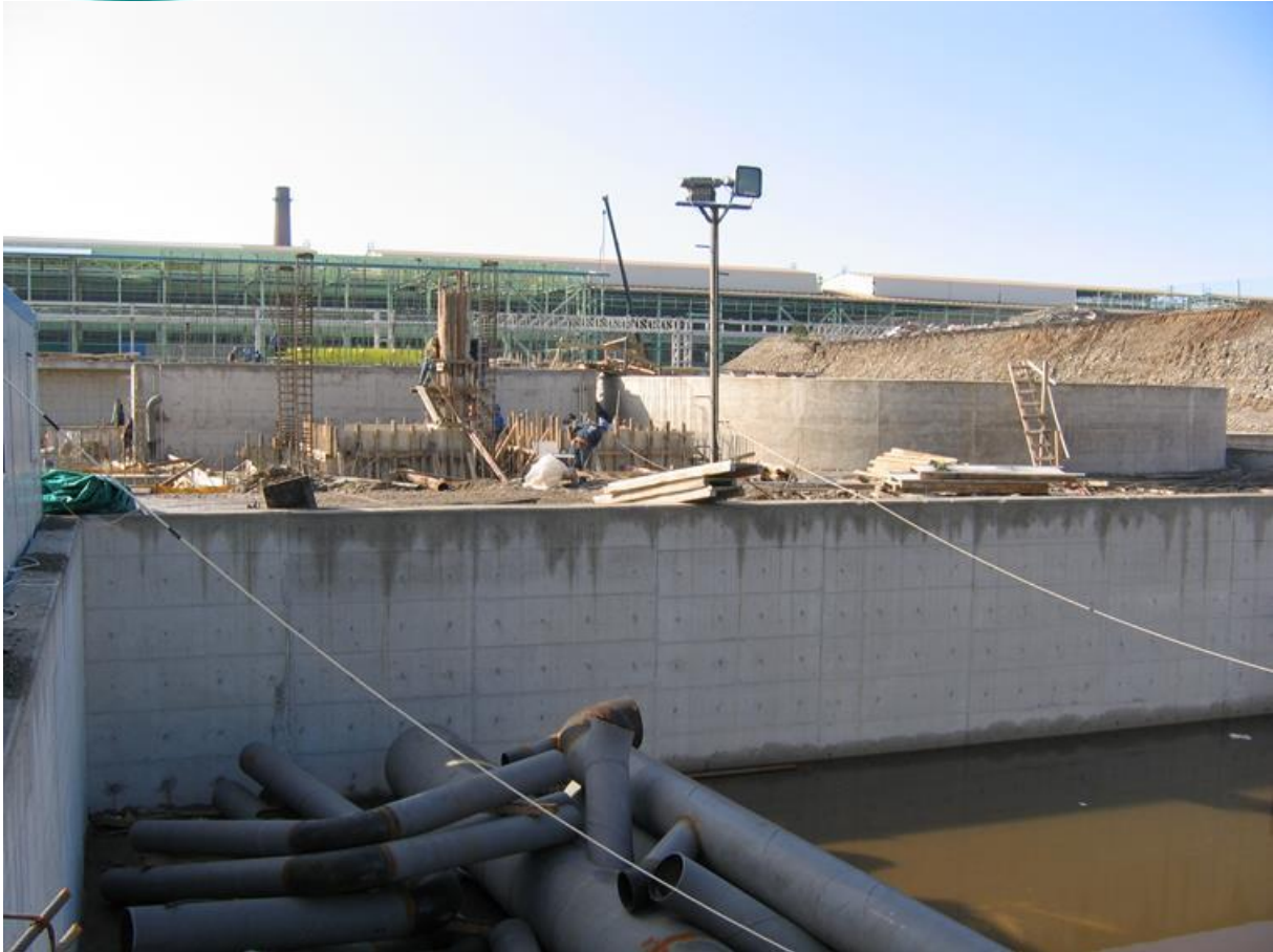
Sludge Thickener Area Construction
