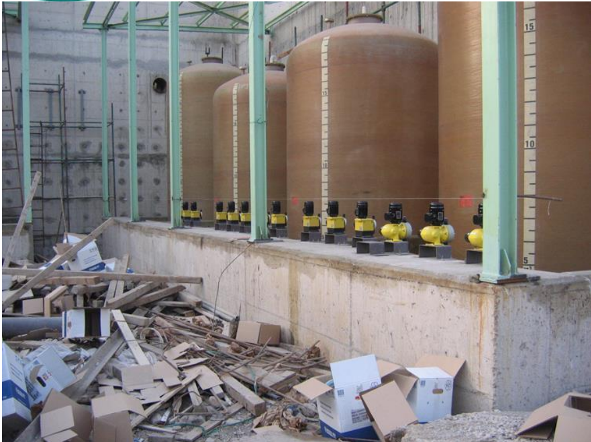
Chemical Dosing Units Construction
