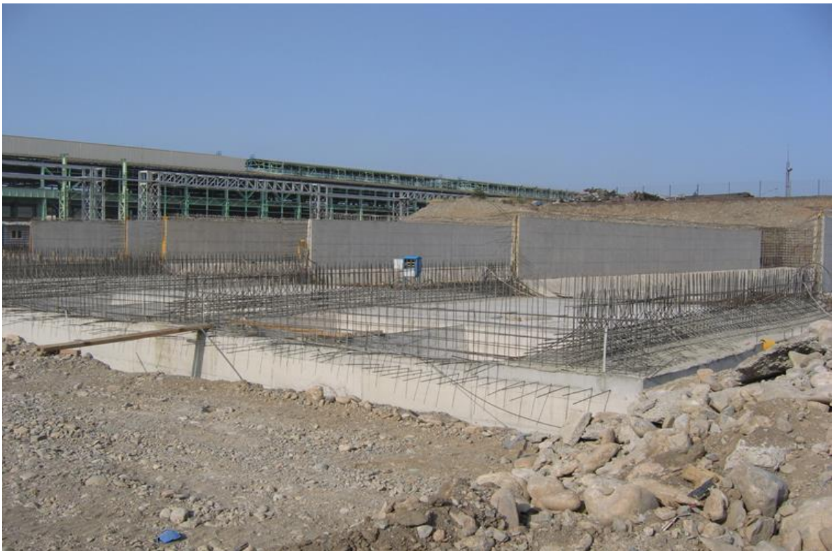
Settling Basin Construction
