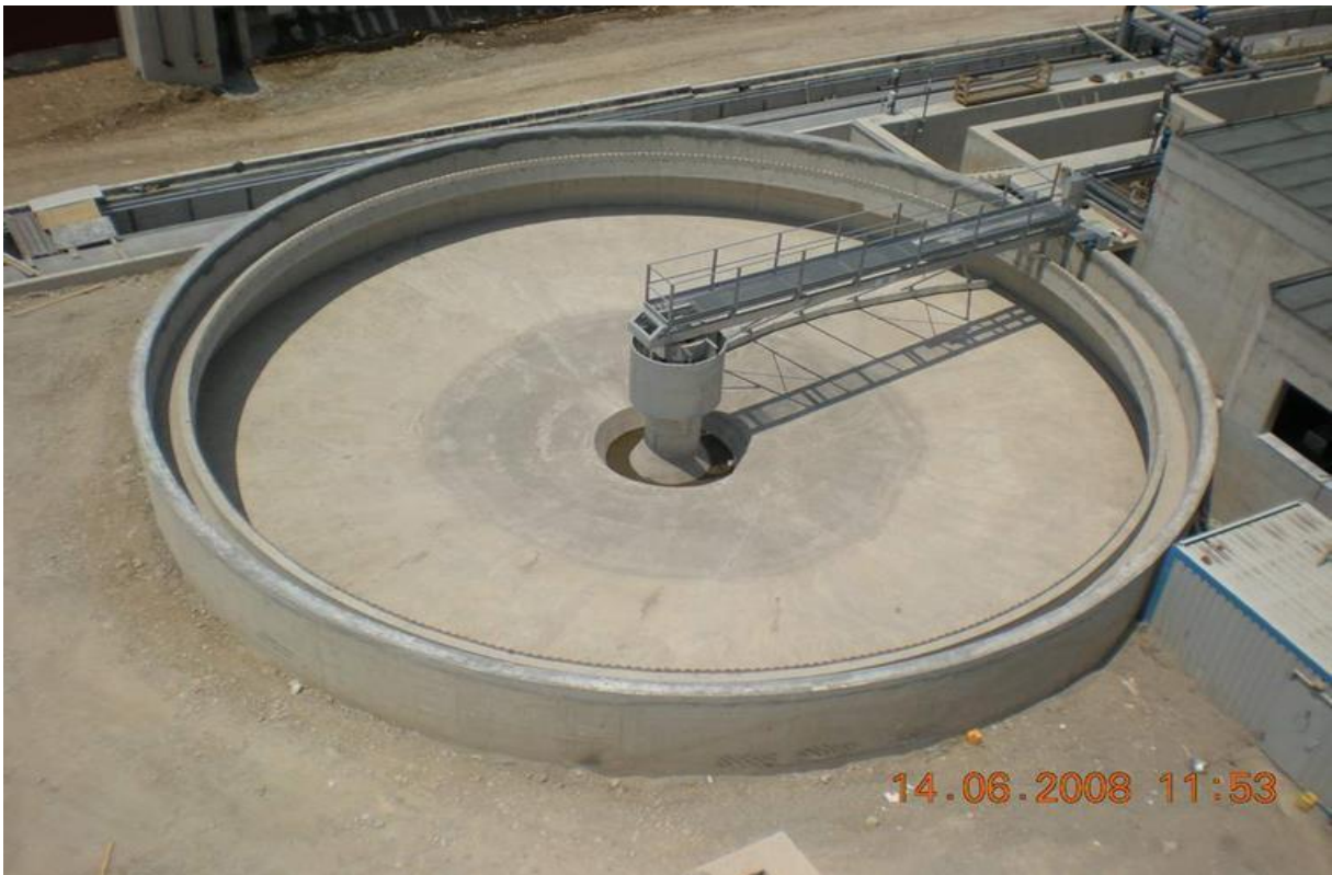
Sludge Thickener Area General Appearance
