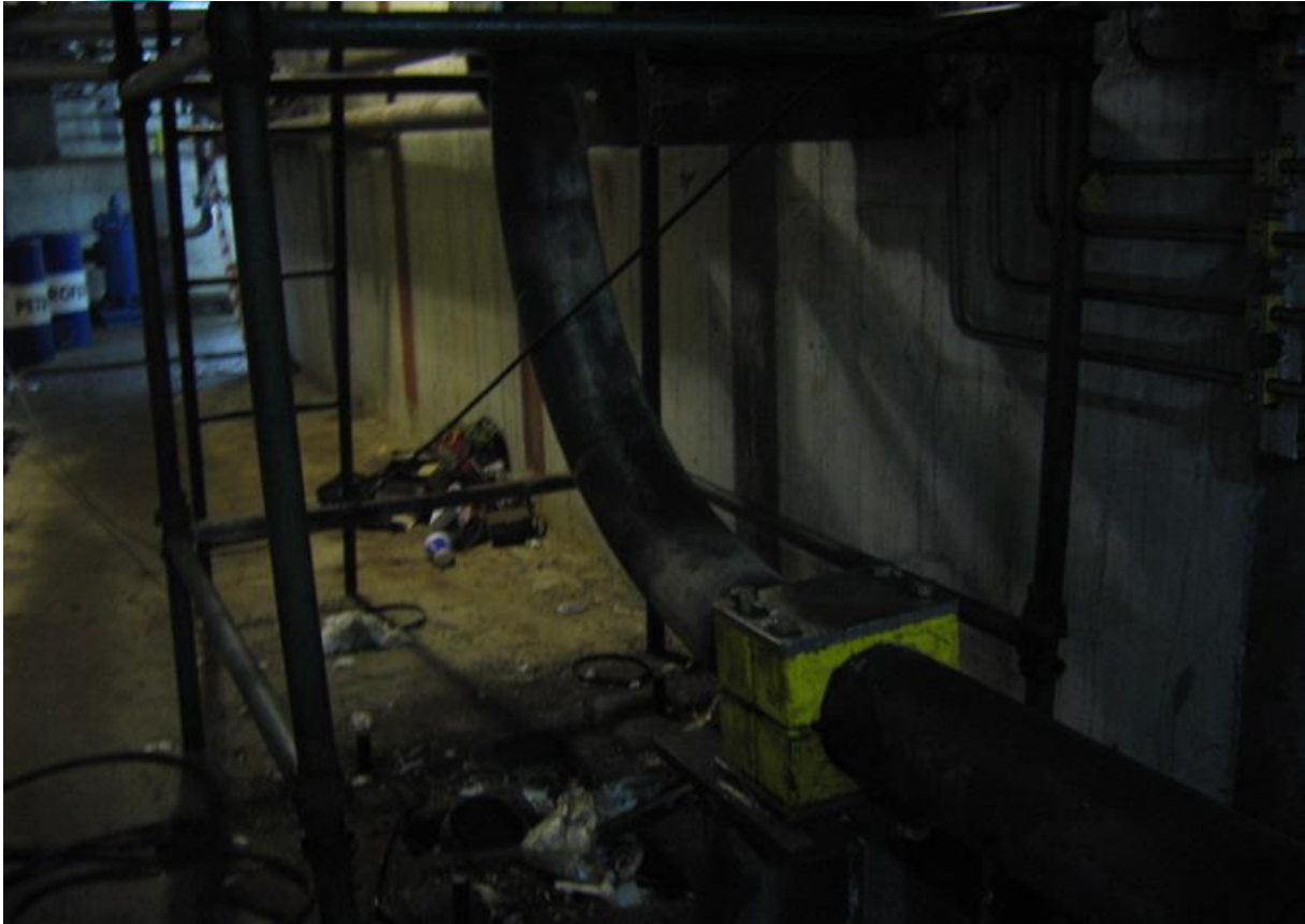
Descale Pump Dicharge Line Generel Appearance
