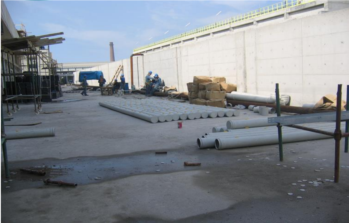
Cooling Towers Inside Distributor Channel Installation
