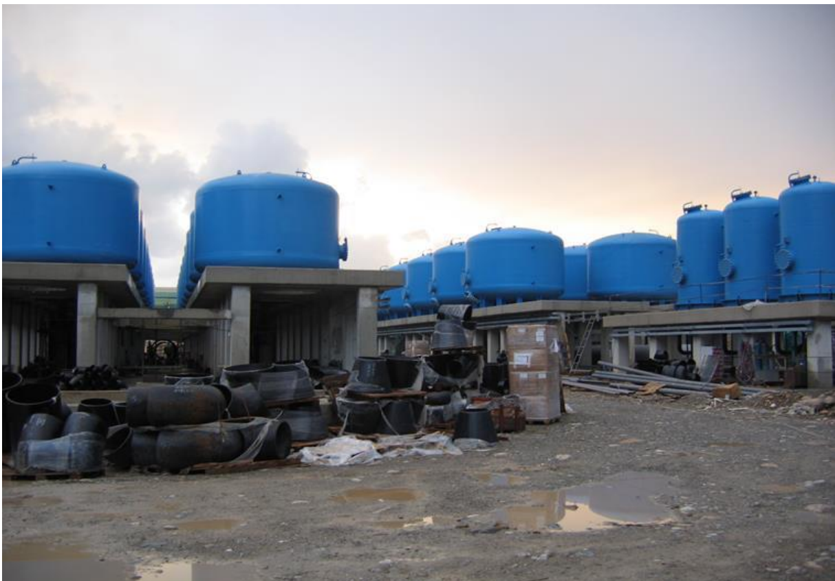
Sand Filter Area Installation
