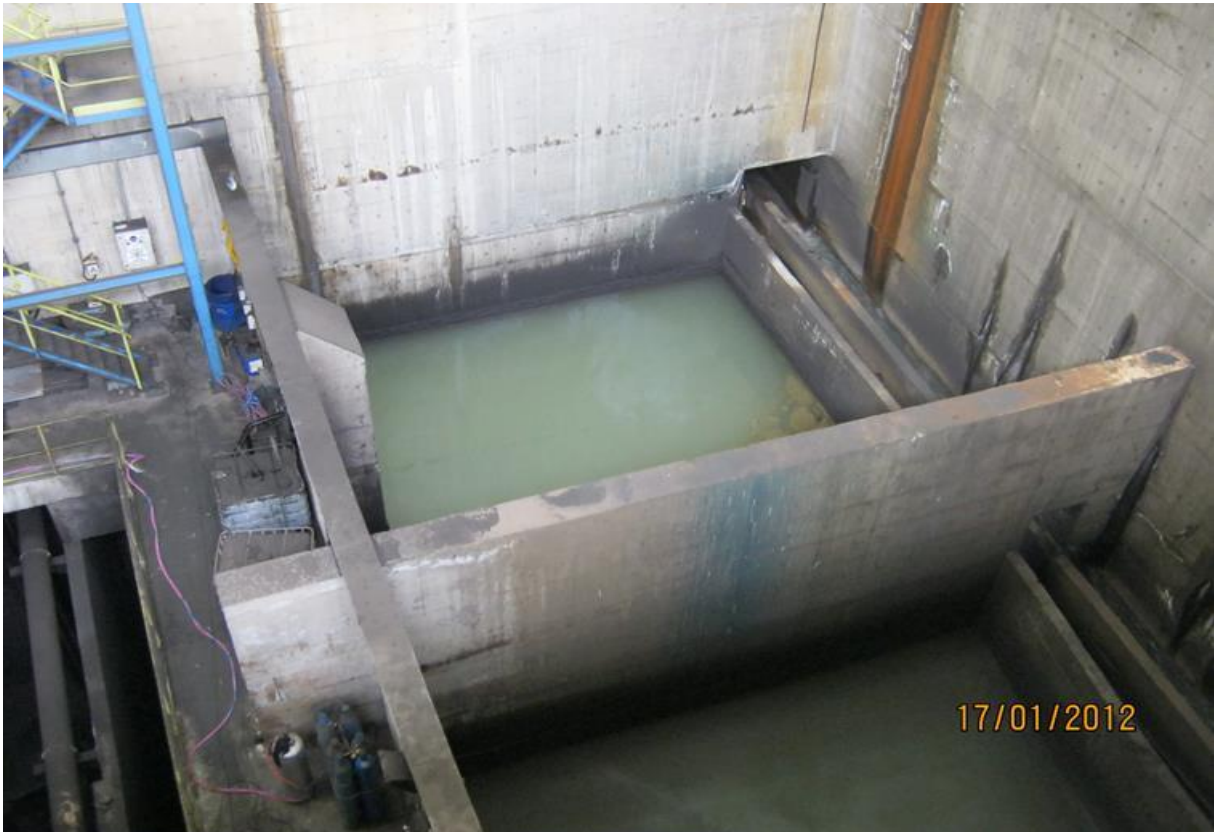
Scale Pit Area
