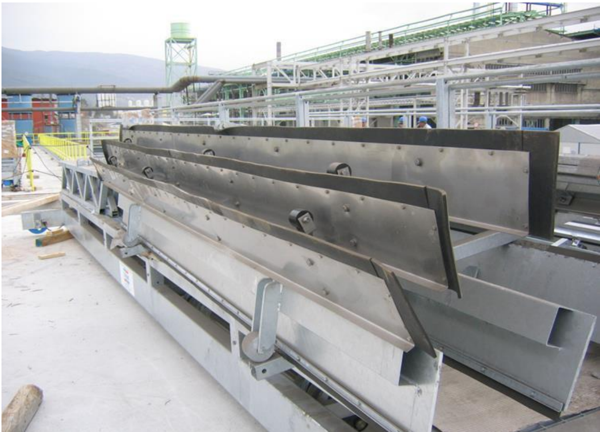
Settling Basin Scraper Bridge Installation
