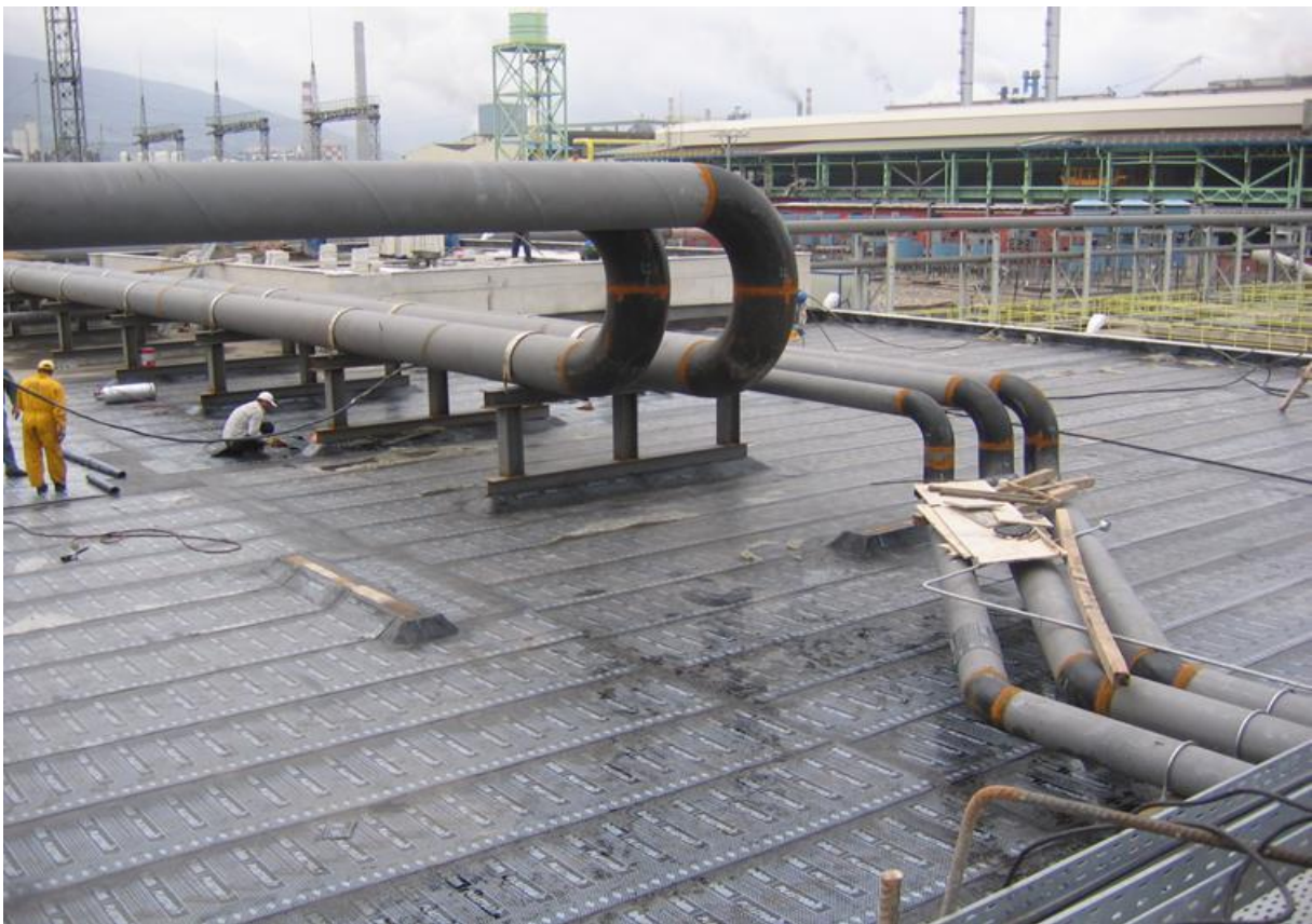
Pump Piping Installation
