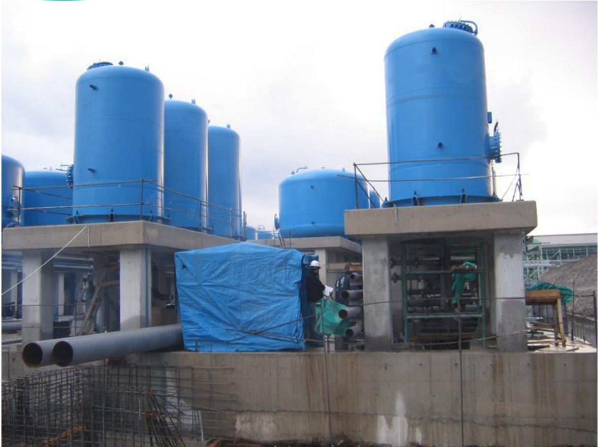
Sand Filter Area Installation
