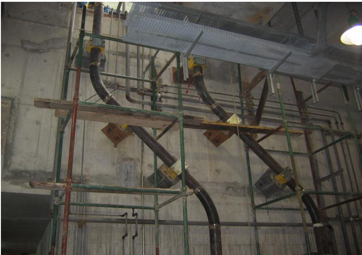
Descale Pump Discharge Line General Appearance
