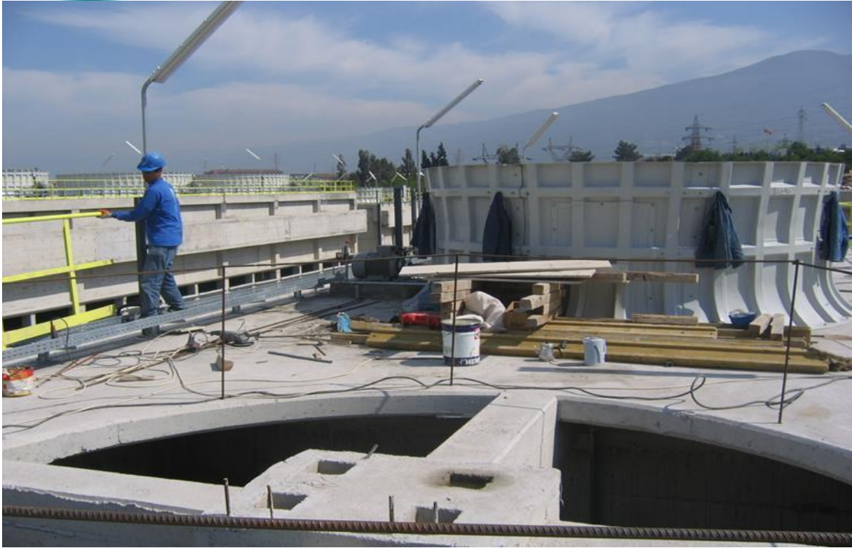
Cooling Towers Installation
