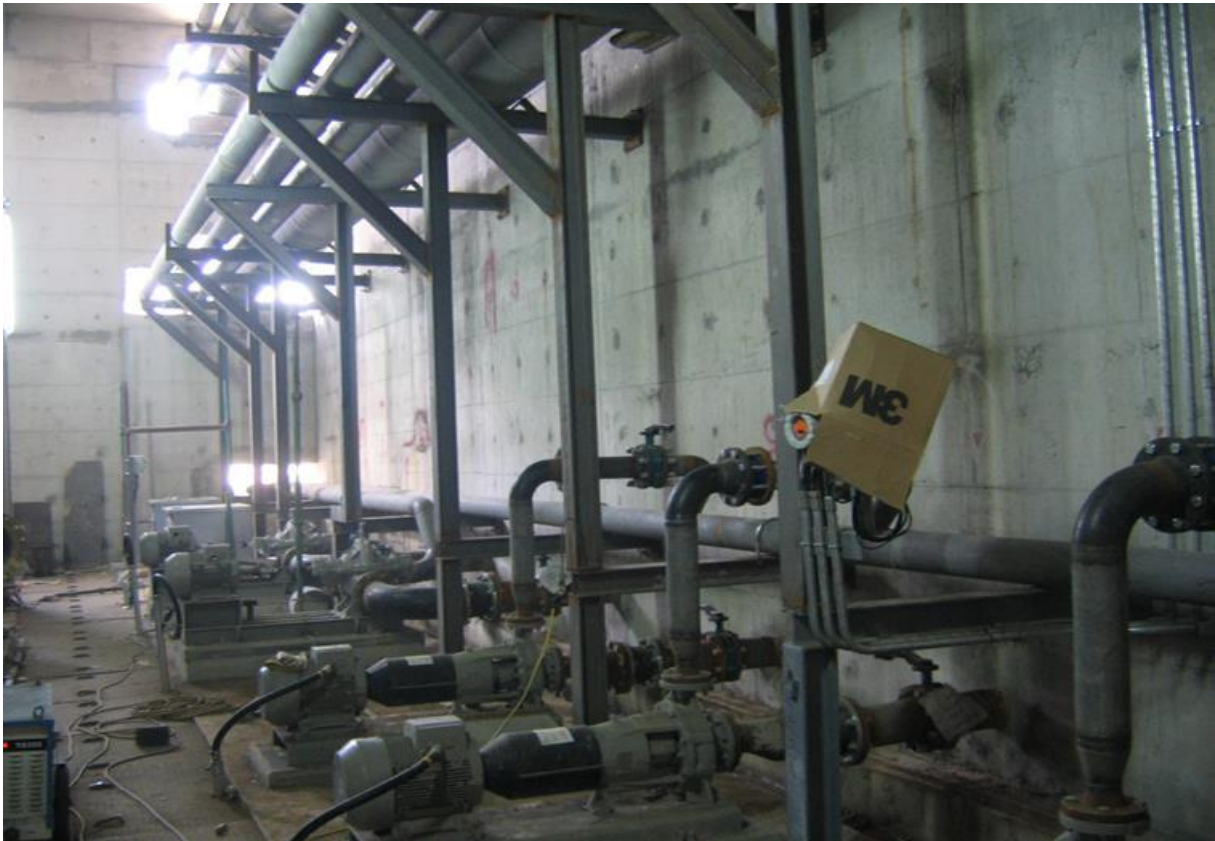
Pump Hall Piping Installation
