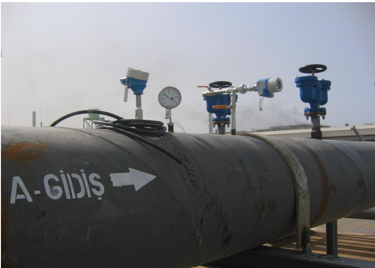
Pump Discharge Line Flowmeter ,Temperature Trnsmmitter, Manometer Installation
