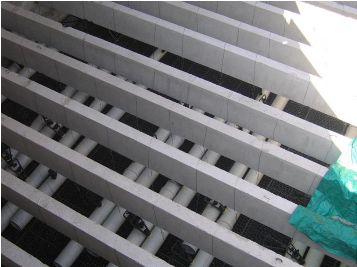
Cooling Towers Inside Distributor Channel Installation
