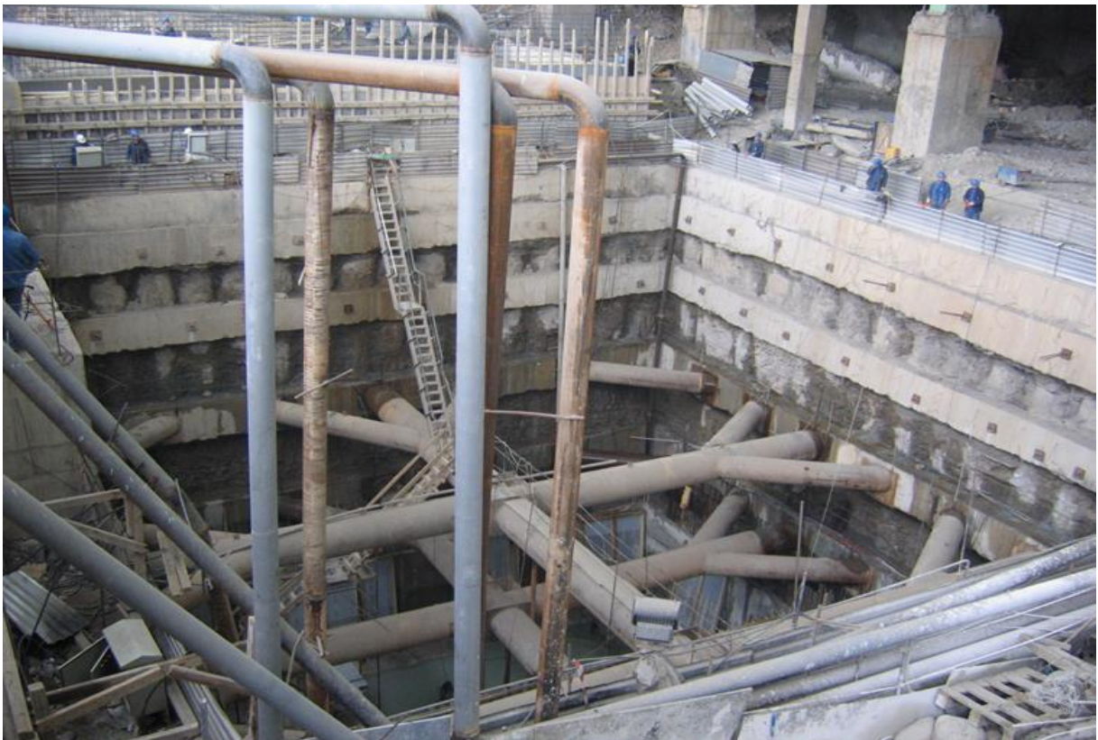
Scale Pit Construction Work
